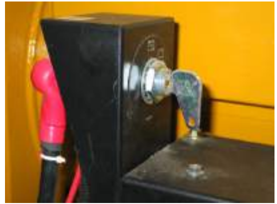
Figure 5-25 Genset Battery Master Key
