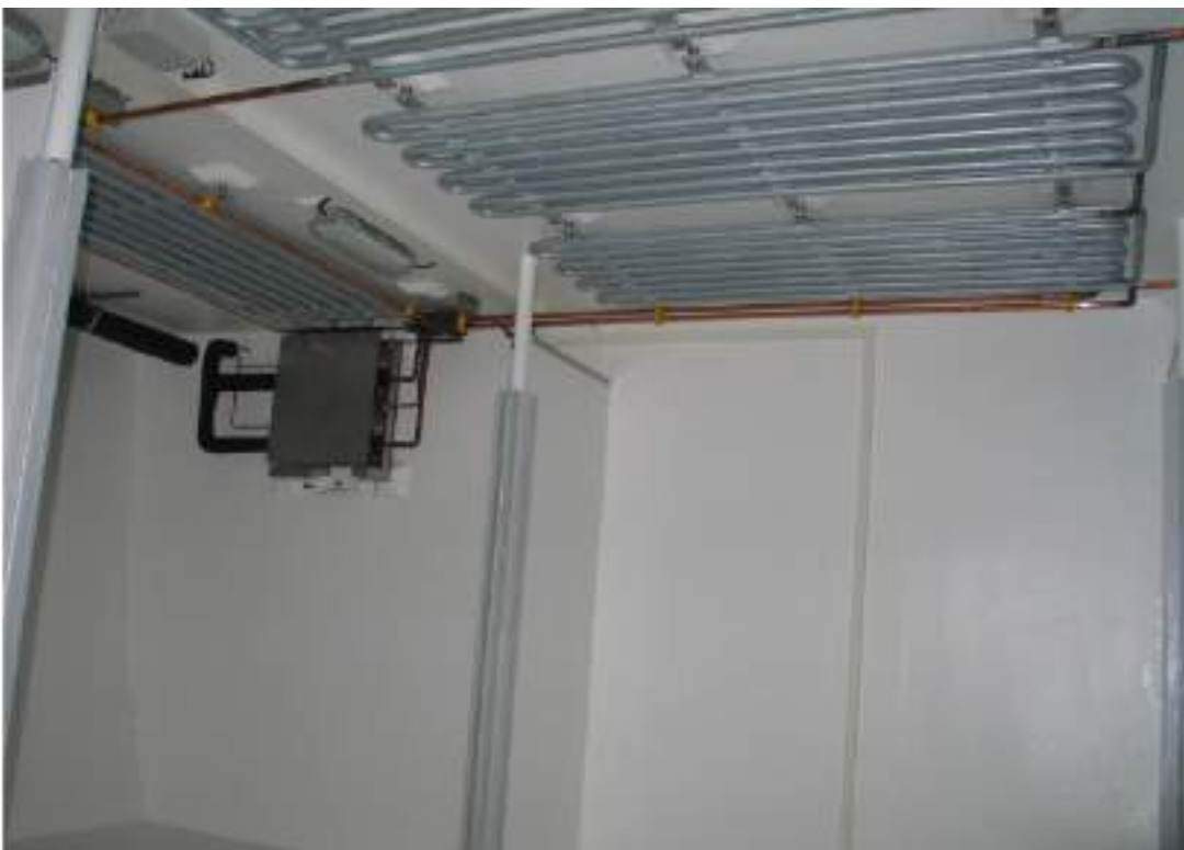
Figure 2-41 Stbd Bulkhead Fish Hold
