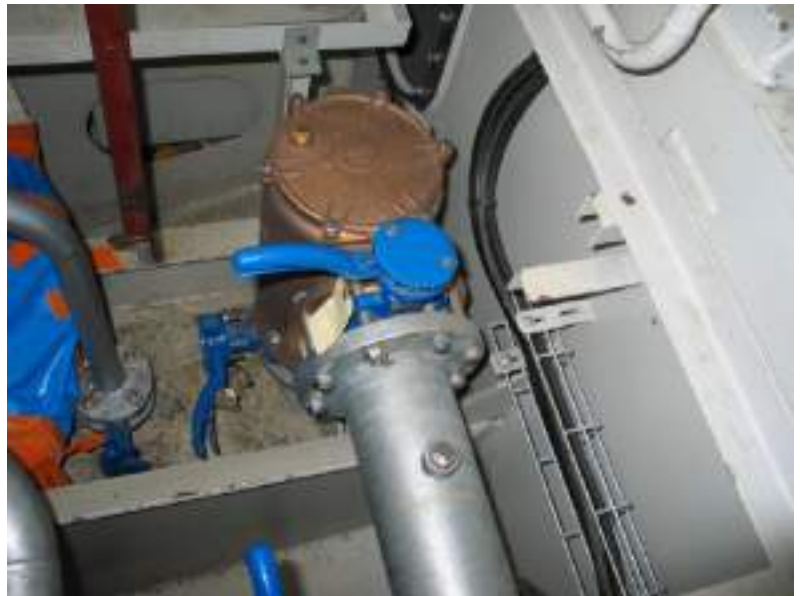
Figure 5-38 SW Strainer
