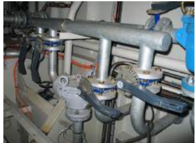
Figure 5-12 Bilge Manifold
