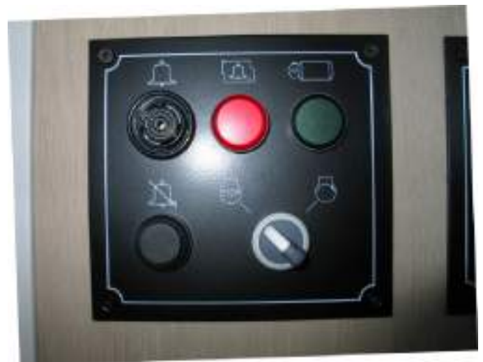
Figure 5-27_Genset Remote Control Panel
