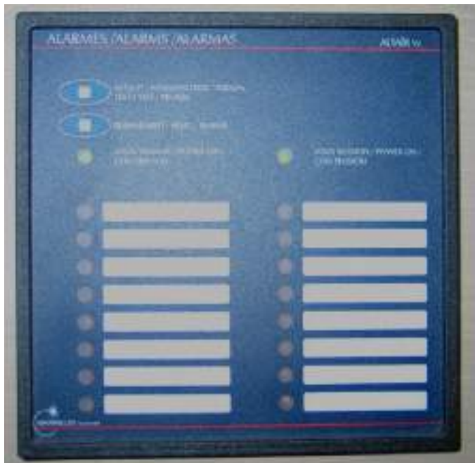
Figure 5-29 General Alarm Panel
