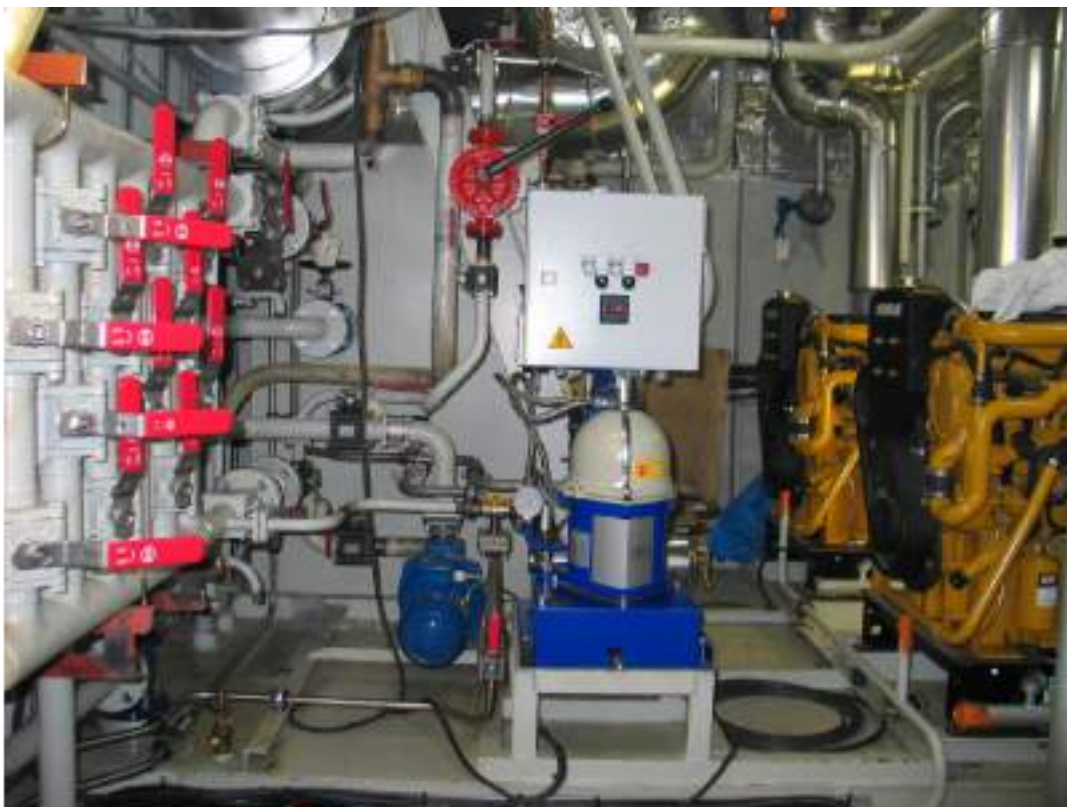
Figure 2-37 Engine Room - Port Bulkhead
