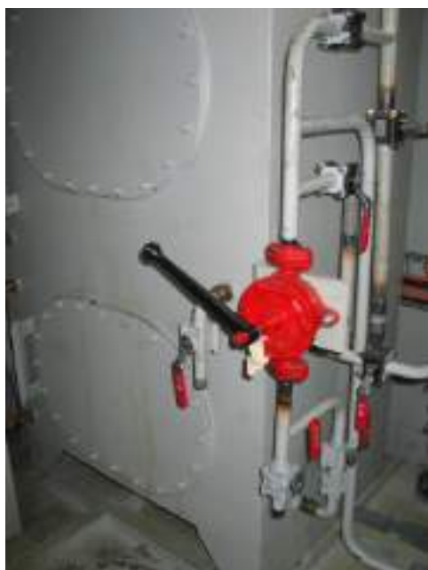
Figure 5-19 Lubricating oil Transfer Hand Pump
