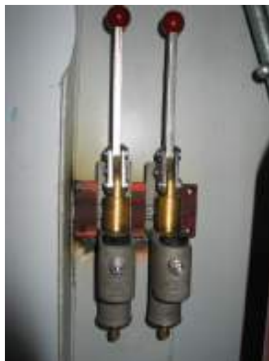
Figure 5-18 FO Quick Closing Valves
