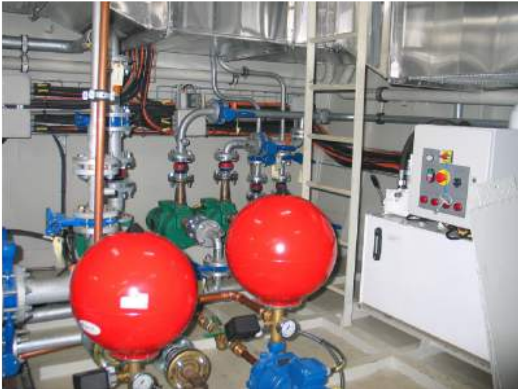
Figure 2-36 Engine Room - Stbd Fwd Bulkhead
