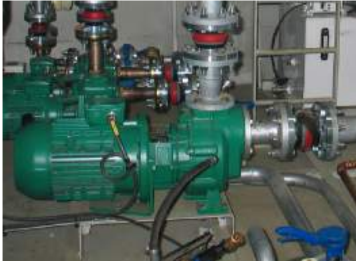
Figure 5-8 Fire Pump
