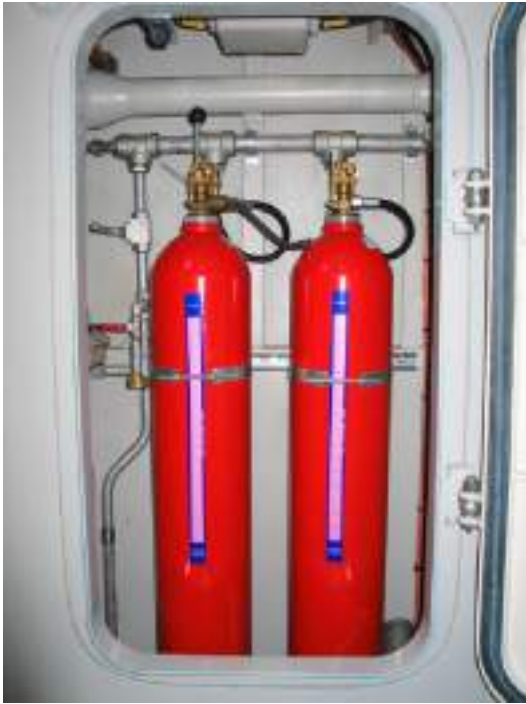
Figure 5-20 CO2 Cylinders 1 and 2
